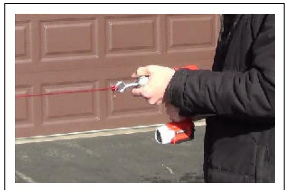
bolt into the chuck of a portable drill, as shown in the last photo here. Next, from the eyebolt, stretch all of the wires back toward the anchor post and re-attach them to the anchor post so that each wire is exactly the same length. You'll see why this is important in the next picture.
